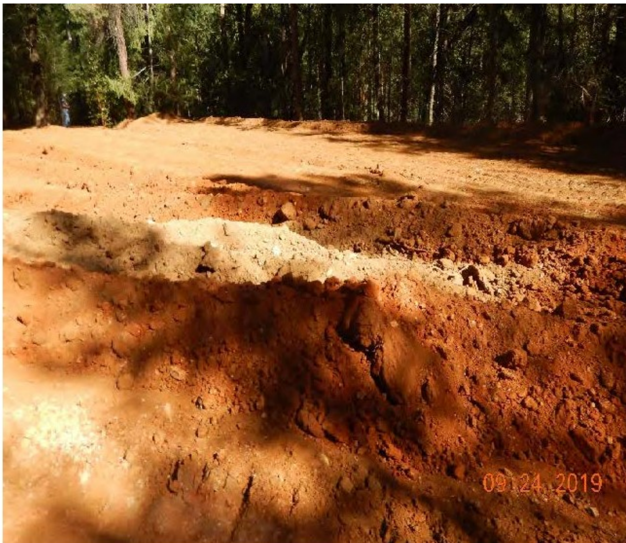
Freshly graded pad along the Northern Access Road.
